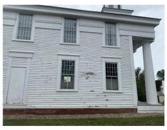
• The cornice molding at the base of the front pediment sags in the center. This is likely due to slippage of the wood furring that supports the cornice and should be monitored.
